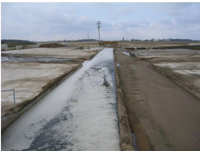
Figure 4–47 Dual sand lanes used to remove sand from dilute, flushed dairy manure (Holmes 2010). One lane is allowed to drain and is cleaned while the other is used to treat manure. Note the location of equipment access ramps and sloped pads for sand conditioning and storage
