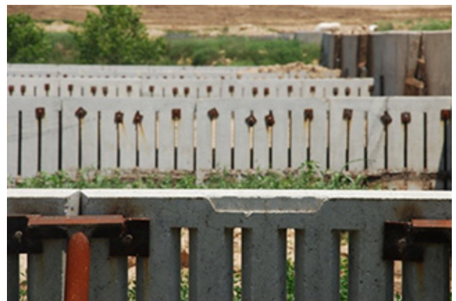
Figure 4–63 Vertical concrete slotted panels provide 1-inch-wide vertical openings (Mukhtar et al. 2011)
