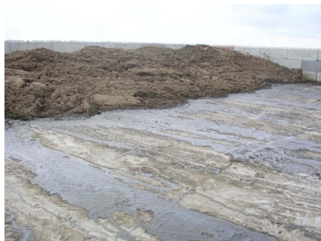
Figure 4–47 Dual sand lanes used to remove sand from dilute, flushed dairy manure (Holmes 2010). One lane is allowed to drain and is cleaned while the other is used to treat manure. Note the location of equipment access ramps and sloped pads for sand conditioning and storage
