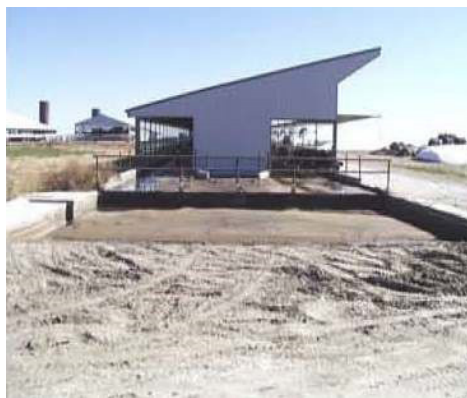
Figure 4-50 Sand trap positioned on the end of a flushed, two-row freestall barn (Wisconsin University, Cooperative Extension & Kansas State University, Cooperative Extension, Harner 2009).
