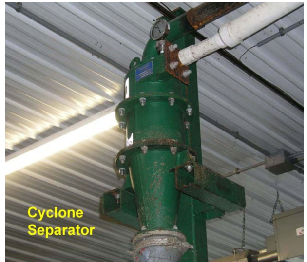
Figure 4–57 A cyclone separator used to remove fine sand from the effluent of a SMS (University of Wisconsin, Cooperative Extension Service, Holmes 2010)
