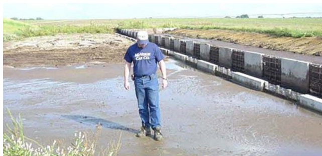
Figure 4–60 Full settling chamber with sand near the fill end (beneath the dairy producer and accumulated dairy solids at the back) (Fulhage 2003)
