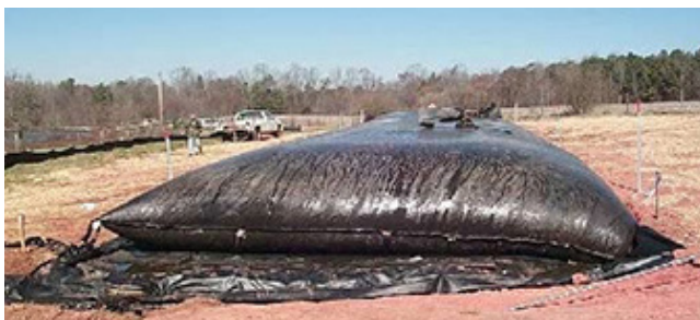
Figure 4–16 Geotextile tube dewatering dairy lagoon sludge (University of Georgia Cooperative Extension)
