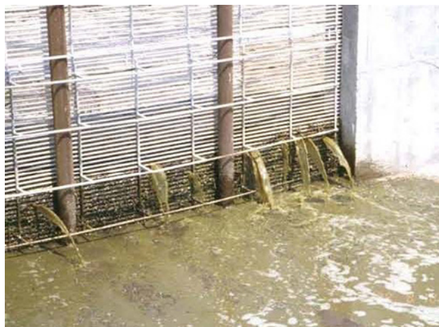
Figure 4–59 Swine nursery flooring panels used to provide the 8 ft. wide porous sections bar spacing is about 3/8 of an inch (Fulhage 2003)
